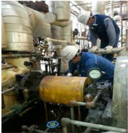
C-P4003B Bearing Jacket Unplugging 작업
