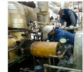
C-P4003B Bearing Jacket Unplugging 작업
